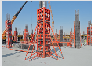
Column Formwork
