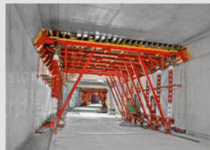
Tunnel Formwork
