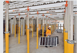
Slab Formwork
