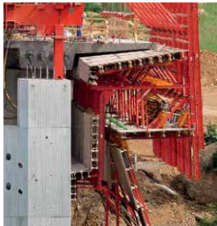
Moving past the piers is possible without any problems after the working platform and slab formwork have been hydraulically folded in.
