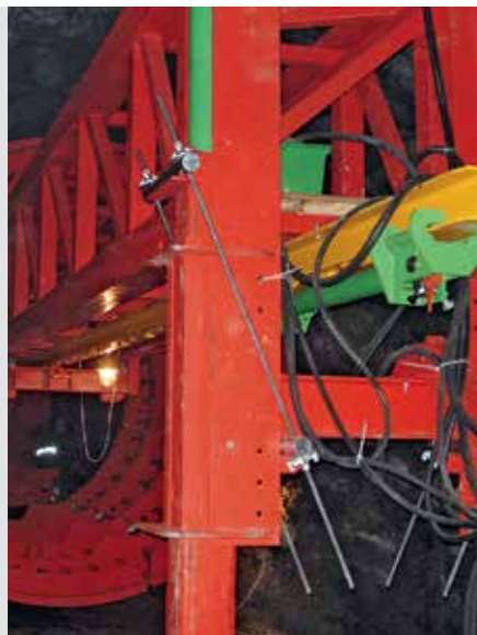
units and hydraulic cylinders for operating the wall and slab formwork elements are available in
