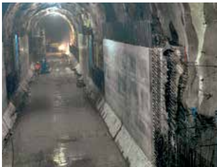
Best concrete results from the 2nd cycle (wall area) form the exit for the arched formwork carriage.
