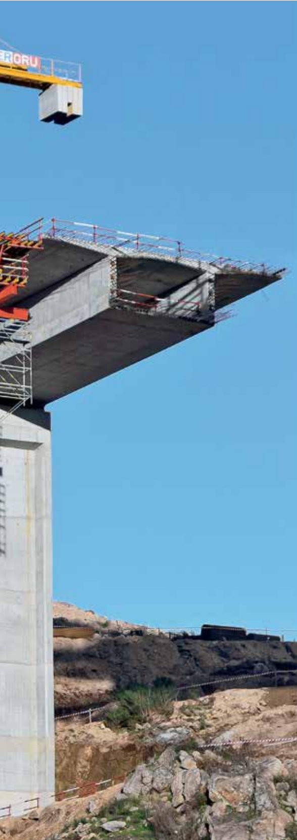
A typical application example in bridge construction. VARIOKIT heavy shoring tower with heights from approx. 5.00 m up to 40.00 m.
