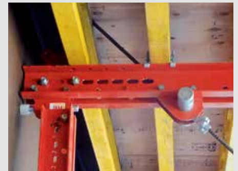
Tie Yoke Head SRU with DW 15 tie rod, can be operated from the underside of the bridge.
