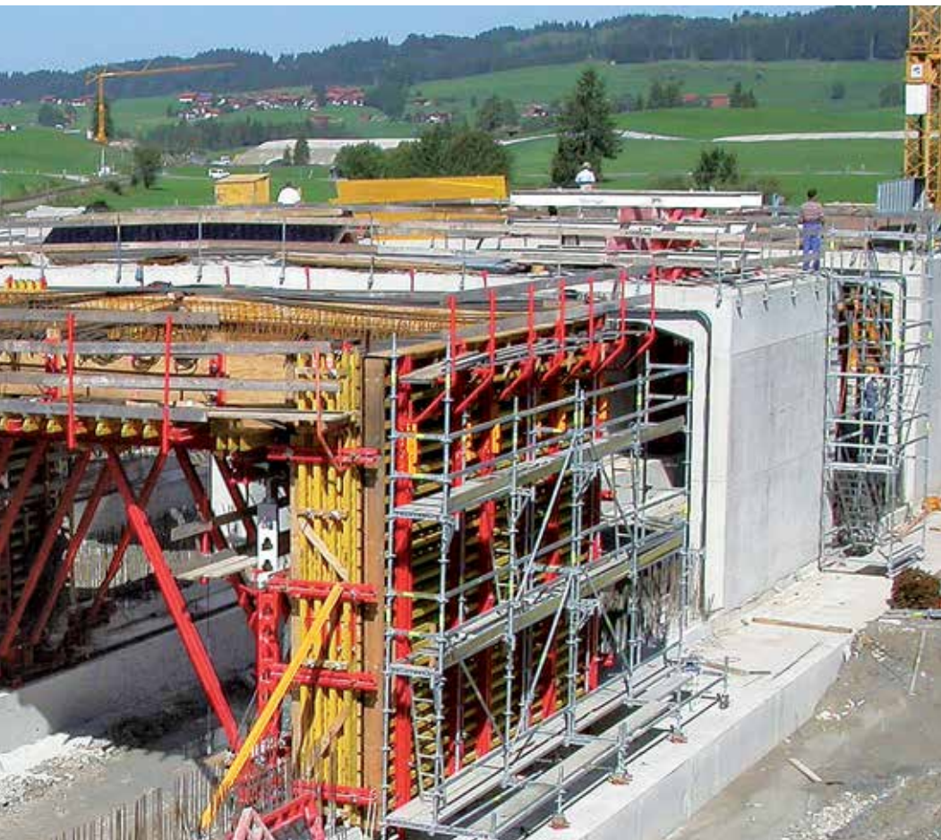
The combination of proven systems such as VARIO GT 24 and HD 200 with new elements from RCS or the diagonal strut, results in a cost-effective formwork carriage.
