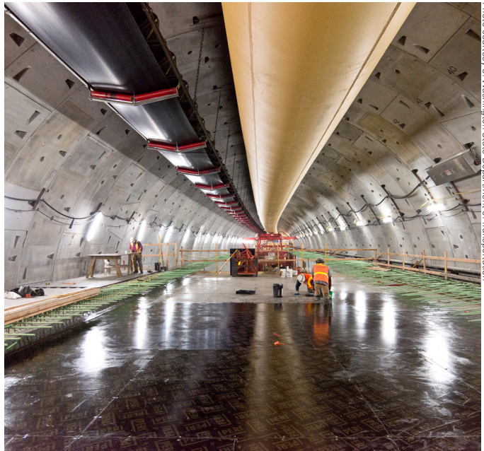
Photo courtesy of Washington State Department of Transportation
