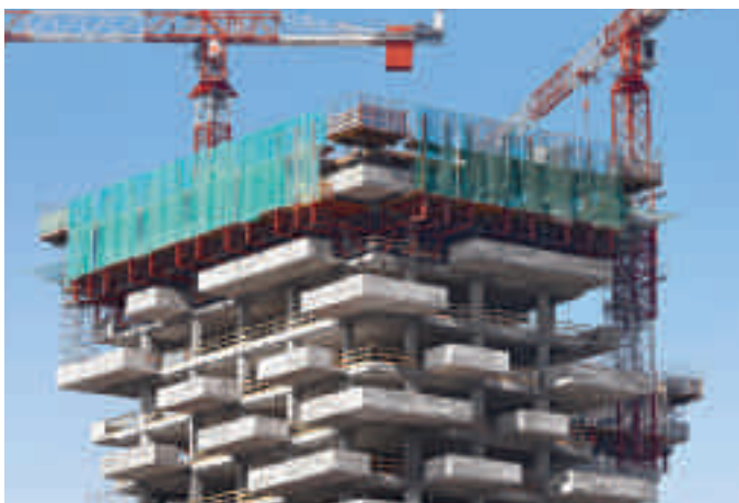
With a 150° rotation, the Evolution Tower twists its way upwards into the Moscow sky reaching a height of almost 250 m. Inclined and crane-independent climbing RCS Protection Panel Units provide a very high level of safety.
