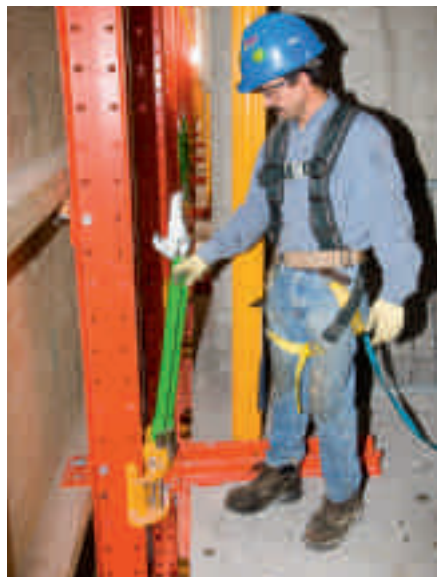
The hydraulic cylinder with its 5 t lifting capacity is positioned on the climbing shoe.
