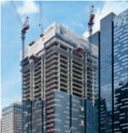
The RCS Climbing Protection Panel in use for the construction of the Asia Square Tower in Singapore. The integrated landing platforms ensure easy transport of materials from floor to floor.
