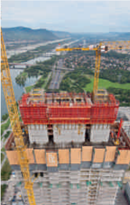
The repeatedly recessed facade construction characterizes the DC Tower in Vienna. The Climbing Protection Panel could be continually adjusted to match the variable floor areas.
