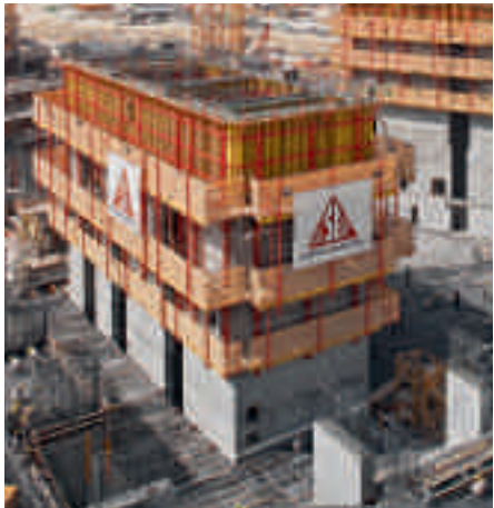
Safe working conditions with continuous lateral and rear protection on and under the RCS C Climbing Formwork.
