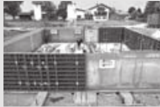
Wall Formwork
