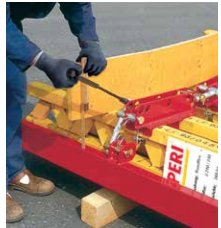
The adjustable spindle for adjusting the edge profile is also operated by means of the "combi" Ratchet Spanner.
