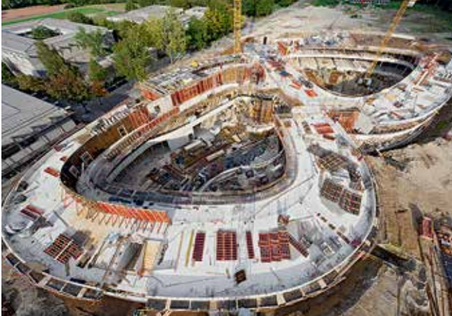
Text-book execution: the in-situ concrete curvatures feature variable radii.
