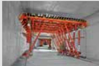
Tunnel Formwork
