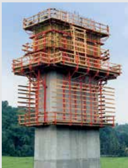
Bridge pier Architectural concrete with CB 240 and VARIO GT 24.
