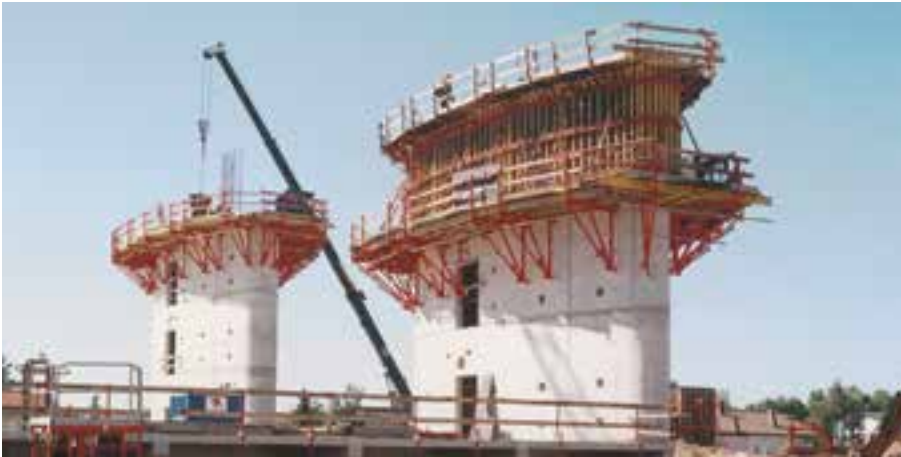
Cultural Buildings High-quality architectural concrete with CB 240 brackets and VARIO GT 24.
