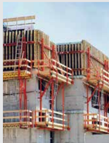
Safety PERI ladder for safe access to the finishing platform.
