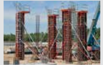
Column Formwork
