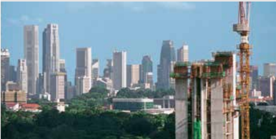
Apartments CB 240 and CB 160 scaffold brackets with VARIO GT 24.
