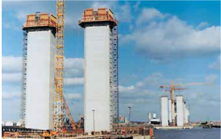
CB 240 with VARIO GT 24 for construction of bridge piers.
