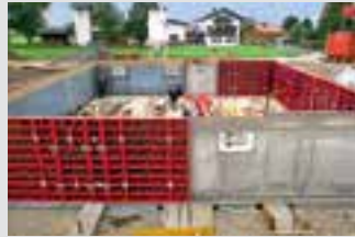
Wall Formwork
