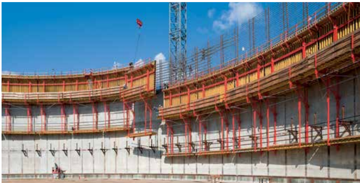
LNG liquid gas tanks Circular walls Ø 77.50 m with CB 240 and VARIO GT 24.
