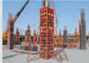
Column Formwork
