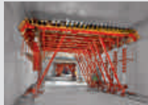
Tunnel Formwork
