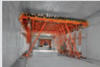
Tunnel Formwork
