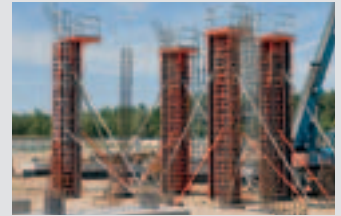
Column Formwork
