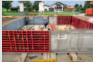
Wall Formwork
