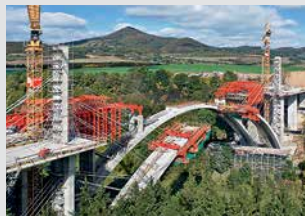
Bridge Formwork
